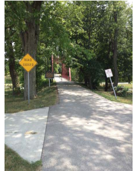
Chinworth Bridge and trail on the west side of Warsaw near Old US 30
